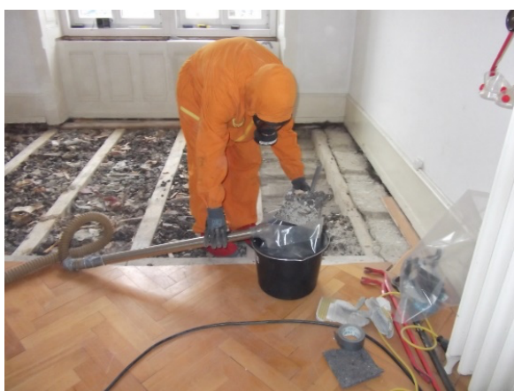
Figure 2 – Remediation work and typical contaminated waste.
